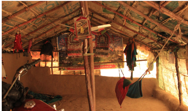
Figure 8. Hut 1 Section. Photographed by Shundana Yusaf.
