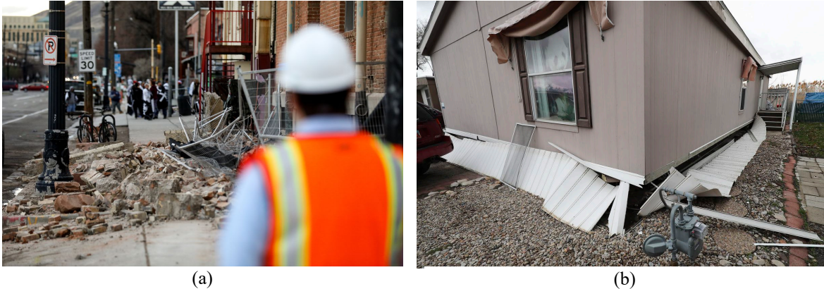
Fig. 4 Images of building damage from the 5.7 Magna Earthquake. (a) Damage to a building in Downtown Salt Lake City. (b) Mobile home in Magna moved off its foundation [7].
